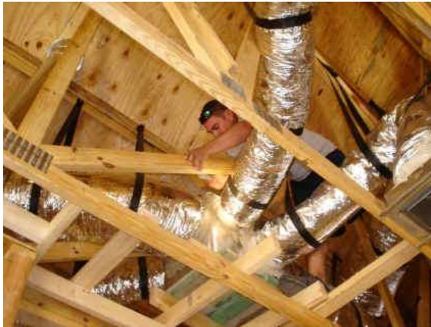
***Duct Technician attending to leakage identified by smoke testing. Failures addressed now, will not be measured as leaks later, when it is too late or too difficult to correct them.***
