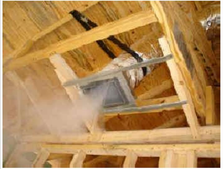
***Most Remote register temporarily unsealed to allow fog to flow through entire Duct System***
